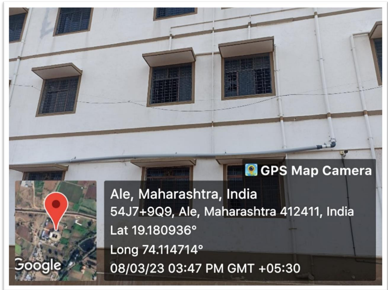
Rain water management system in institute
